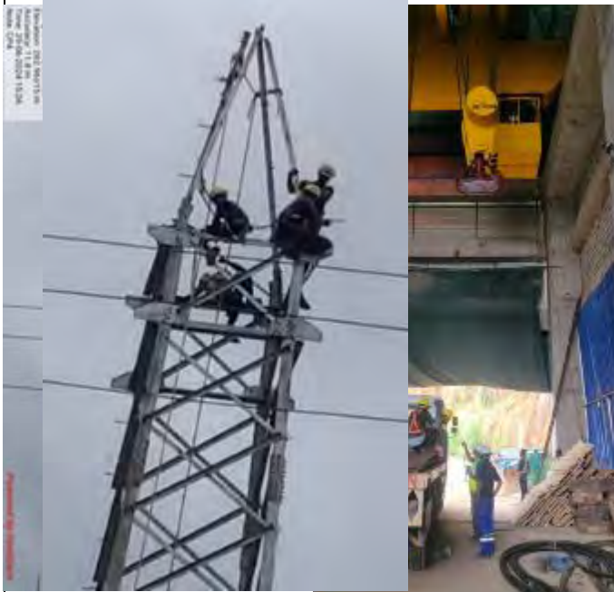
Unsafe working: Worker without PPE's and workers standing below the Crane Pulley
