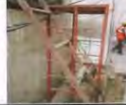
Non-standard laddar engaged in job unit-2.
