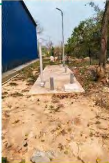
Septic tank at the back side
