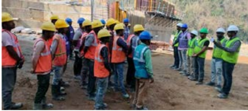
Onsite Training – Construction Safety Measures
