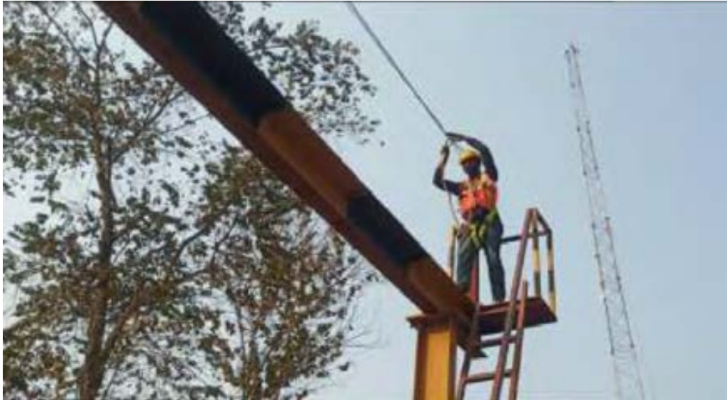
CP-4. Height pass issues to all the tower workers
